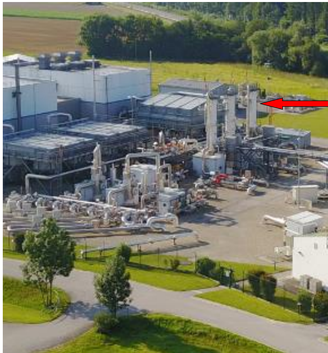
Underground gas storage facility with glycol dehydration units
